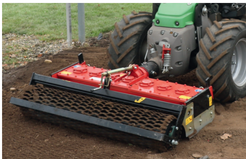
The result: levelled and finely loosened ground with a compacted layer of top soil
